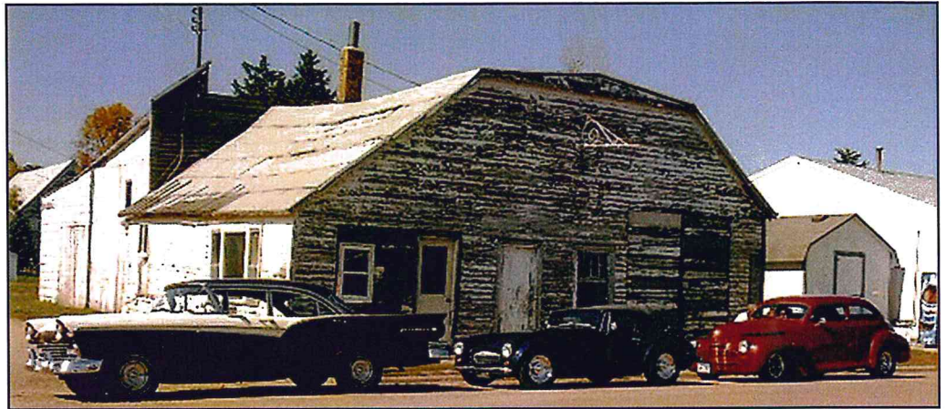
STORAGE SPACE – Don Jensen reportedly bought this place for future storage, and some of the Great Plains Streetrodders stopped by to scope it out, maybe wanting to store their cars there this winter. Yeah, it needs a little work, but the rumor is Don has plans that will make this location in Montrose look brand new.
